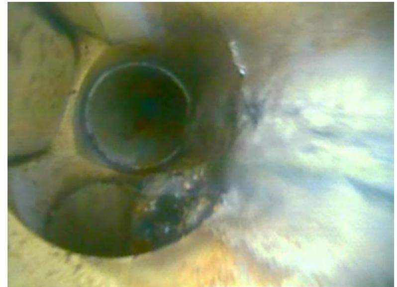
*ABOVE two snapshots from the 'drain cam' movies showing clear drains and junctions.
