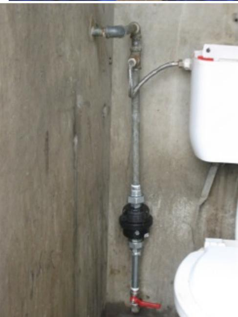
**Water in** — The water was turned off to the local area, the main water supply pipe to each toilet / tap was cut, new pipe and fittings were made to install an isolation valve for water control and a water meter to record use. Because of the high demand on each toilet, the existing toilet cistern was reconnected in the short term, and the mains water turned on to allow use.
